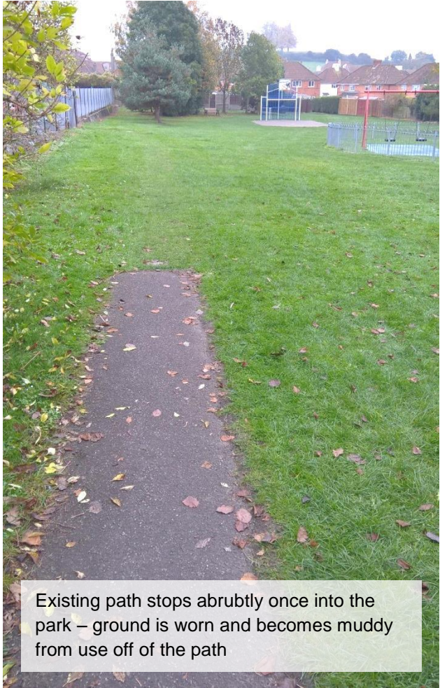
Existing path leading into the park is not wide enough creating muddy strips on either side
