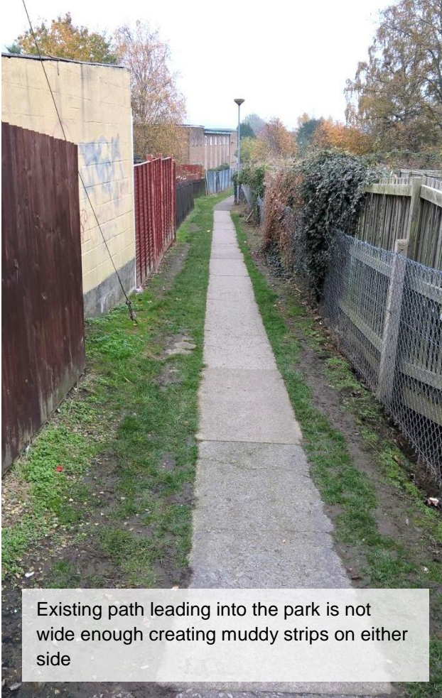
Existing path stops abruptly once into the park – ground is worn and becomes muddy from use off of the path
